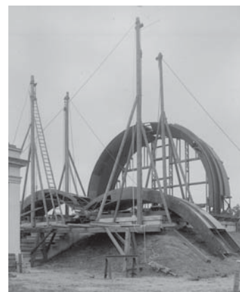
Figure 7. The construction of the domes for the meridian circle in Bergedorf, 1908. 20
