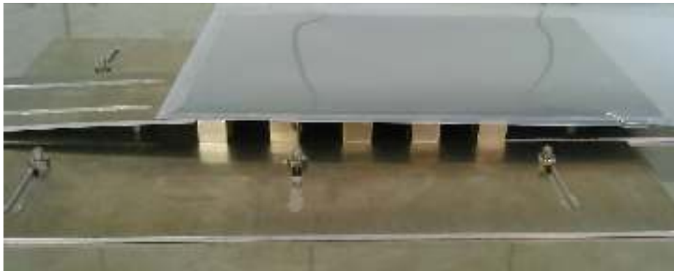
(b) stripes in rail capped with an iron plate before being pushed together
